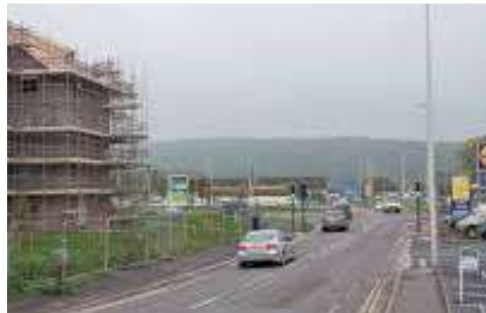
Repairs to Winterstoke Road Bridge are expected to begin in 2022.
